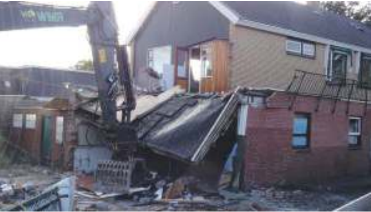
De sloop is in volle gang.
